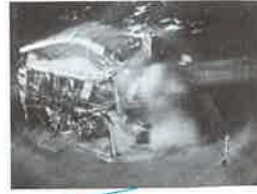
The "after" blast photographs showed these suburban houses engulfed in flames and blown to bits within two seconds of being hit with a nuclear bomb.
